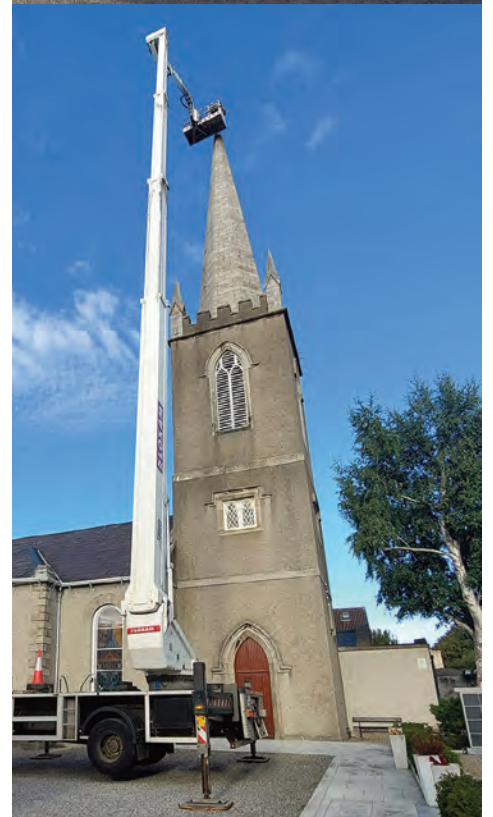
Recent steeplejack inspection of cracks in the spire.
